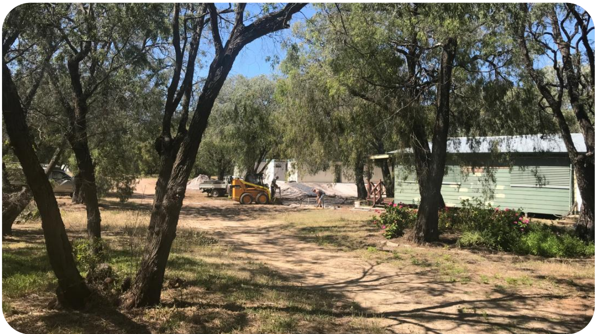
The Family Reunification Centre in Busselton under construction.
